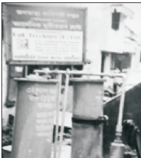
(Fig. g.- i.) Different types of filter plants in public and private places used to remove Arsenic from underground water.
